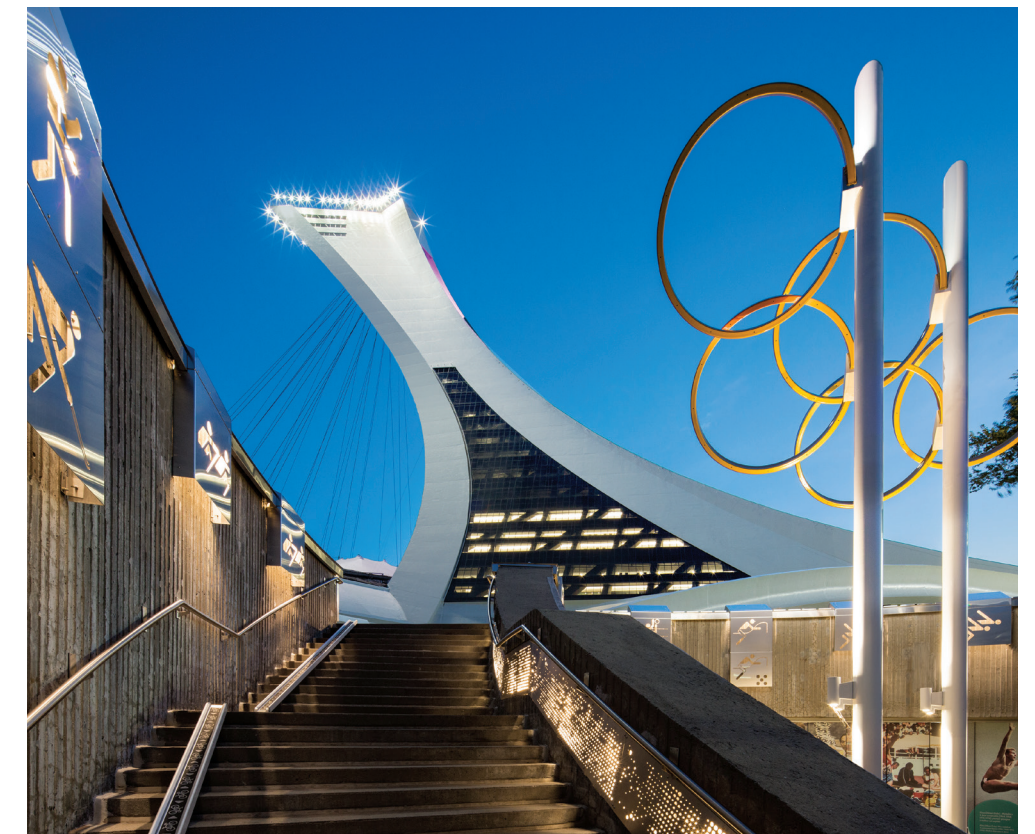
The Olympic stadium's retractable Kevlar roof is supported by cables that hang from a futuristic, swooping tower. The 541-foot-tall structure now houses corporate offices on its unique triangular floor plates, which get smaller as they rise.
