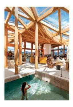
These pages: the main house of the Selva Alegre Residence is roughly 450 square meters in a hexagon like shape. The profile is approx. 20 meters x 20 meters with the center of hexagon approximately 24 meters wide. Heights range from 3.5 to 6.5 meters tall. The wall and roof structures were made from European Spruce.
